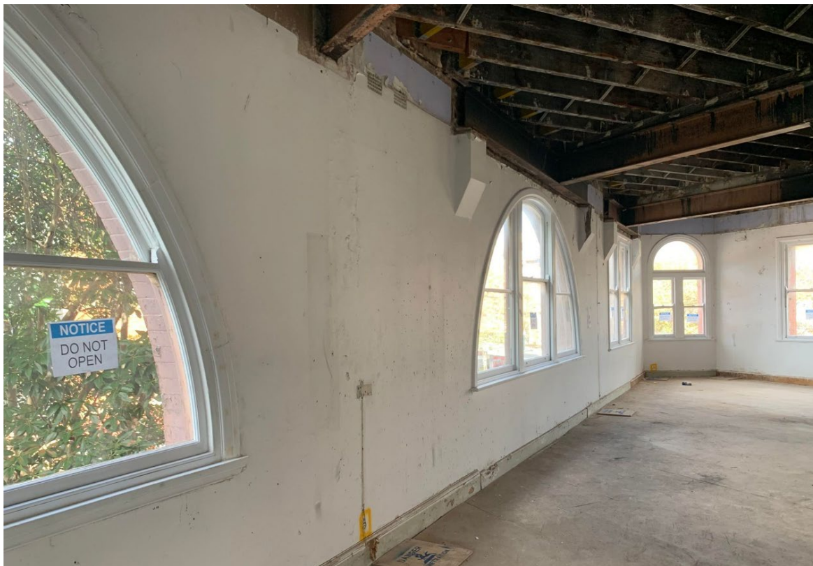
internal view of level 2 of the subject building looking north-west
